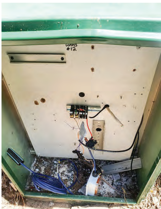
Damage caused by mindless vandalism.
