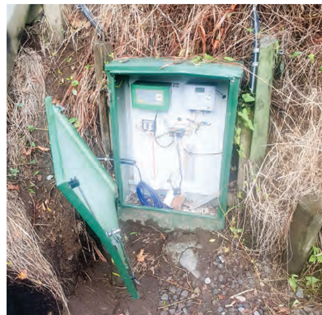
Another image of senseless vandalism.
